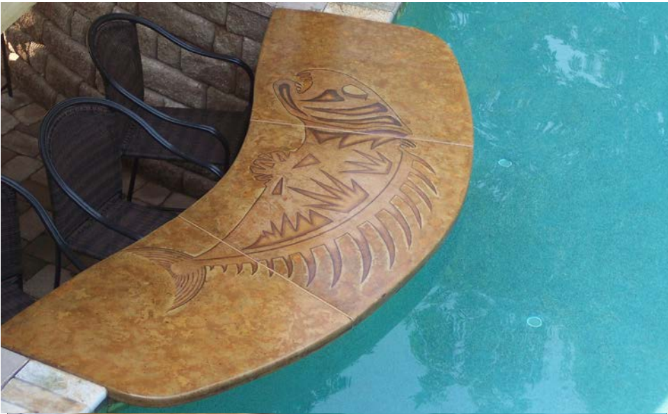
English Red Acid Stain and Coffee Brown Deco Gel Acid Stain (Photo Courtesy of S. Turfle)
