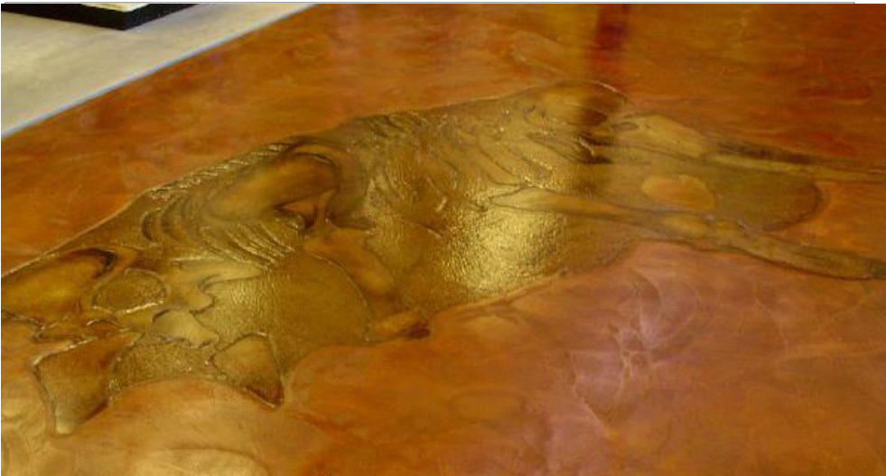
Cola and Coffee Brown Concrete Acid Stain (Photo Courtesy Southeasten Building Maintenance)
