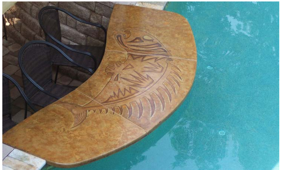
Swim-up pool bar countertop colored with 1311 Concrete Pigment, English Red Acid Stain and Coffee Brown Deco Gel (Photo Courtesy of Susan Turfle)
