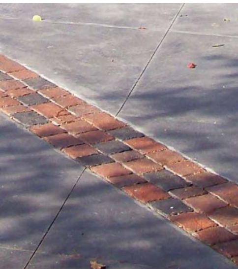
Close-up of stamped concrete walkway as shown above (Photo Courtesy of Decocrete)
