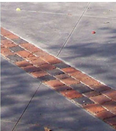
Close-up of stamped concrete walkway as shown above (Photo Courtesy of Decocrete)
