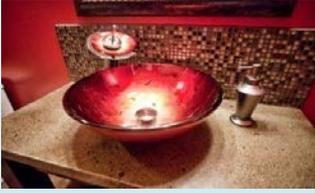
Concrete Acid Stain is a water-based liquid bearing minerals and acid. The acid stain penetrates the pores of the concrete forcing a chemical reaction between the muriatic acid and the available lime in the surface. Once acid stained, the color of the concrete is permanently altered. When sealed with an appropriate concrete sealer and for indoor applications, sealed and waxed, acid stain produces the unique, variegated finish associated with this process.
